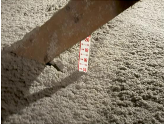
BE1 — 14 inches of blown insulation in the Chapel attic
