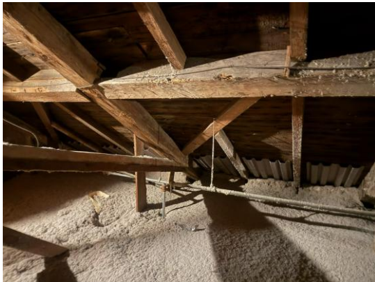
BE2 — Insulators preserved the airflow in the attic by installing baffles around the perimeter.
